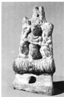
7 Relief of a negro treading an Archimedean screw. The screw thread is set inside a pipe and the negro treads the steps which rotate the pipe and raise the water. Vines are depicted in the background. From Alexandria, first century BC.
