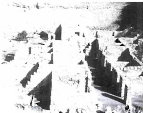
**129 Alexandria (Kom-el-Dik), the townhouses.** The block of houses consists of two ranges of modest units facing each other across a central axis. It was built in the third century and shows some affinities with the apartment-blocks at Ostia in Italy, but differs in being built of local limestone rather than brick.
