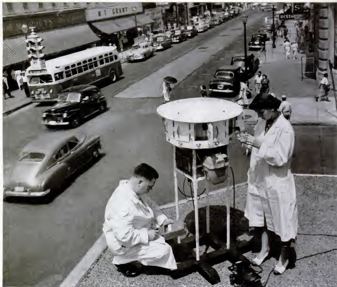
SAMPLING AIR 20 feet above Savannah's Broughton Street, two U.S. Public Health scientists remove flasks filled with germ-trapping broth from experimental sampler atop a store marquee. Sampler has 12 flasks, and air is sucked automatically into them one at a time, 20 minutes each, thus revealing any change
