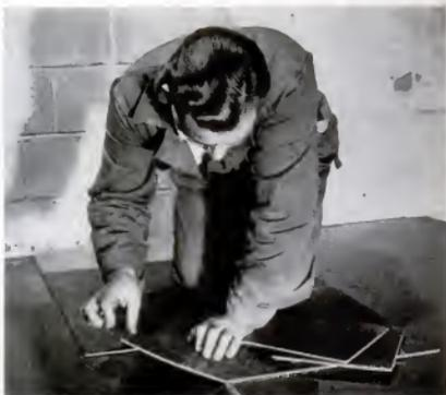
**LAYING CORK TILES** on 20-by-20-foot concrete cellar floor, householder uses six gallons of N-700, which is an easily applied adhesive for any type tiles.
