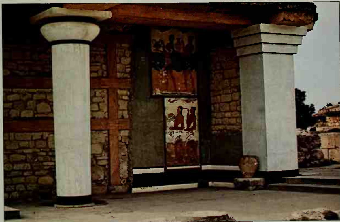
The south anteroom is one of the most thoroughly restored portions of the palace: rebuilt walls, new columns and a fresco in place.
