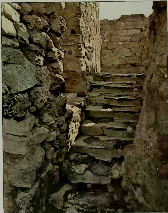
The many staircases at Hagia Triada, like this narrow flight, were built of superbly cut stones, which are in excellent condition even today. These steps descend from the central court level to an area devoted to workshops and storerooms.
