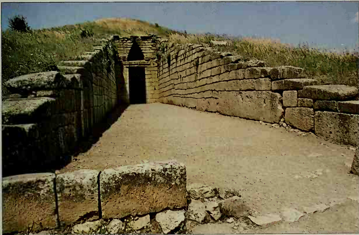
A walled footpath, or dromos, leads to a massive door that is the entrance to the Treasury of Atreus, buried in a hillside at Mycenae.
