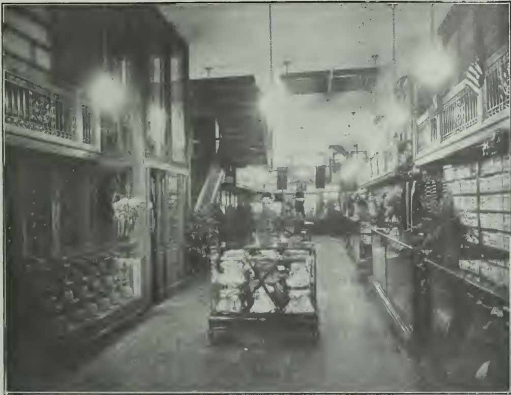
Interior view of the new Allan store, Montreal. Reserve stocks are kept immediately above departments and are accessible by means of a balcony.
