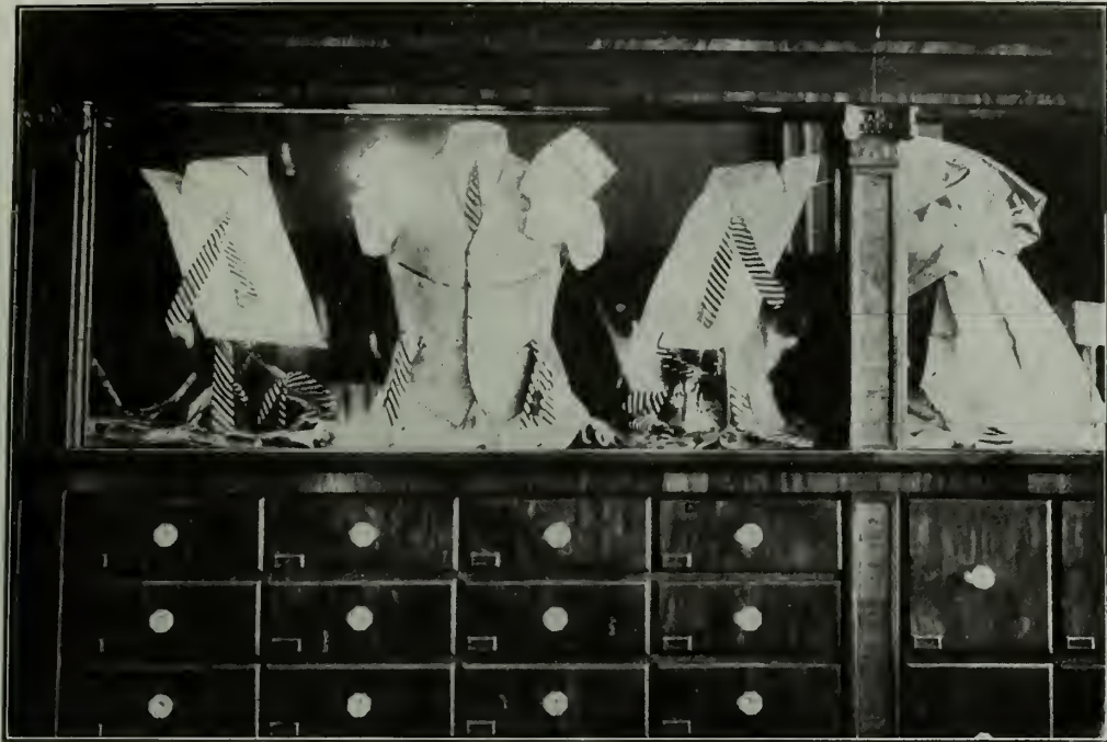
Sectional ledge trim in new Picard & Picard store, Montreal. This haberdashery de luxe is finished in Circassian Walnut and this view also shows the arrangement of stock drawers.
